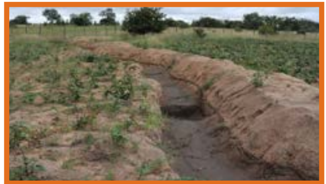
→ A bioswale and infiltration pit that managed to harvest some winter rainwater at Wickrafu Mapfumo's RD site in ward 15 Buhera. © Juliet Madhuku/Takunda RFSA
