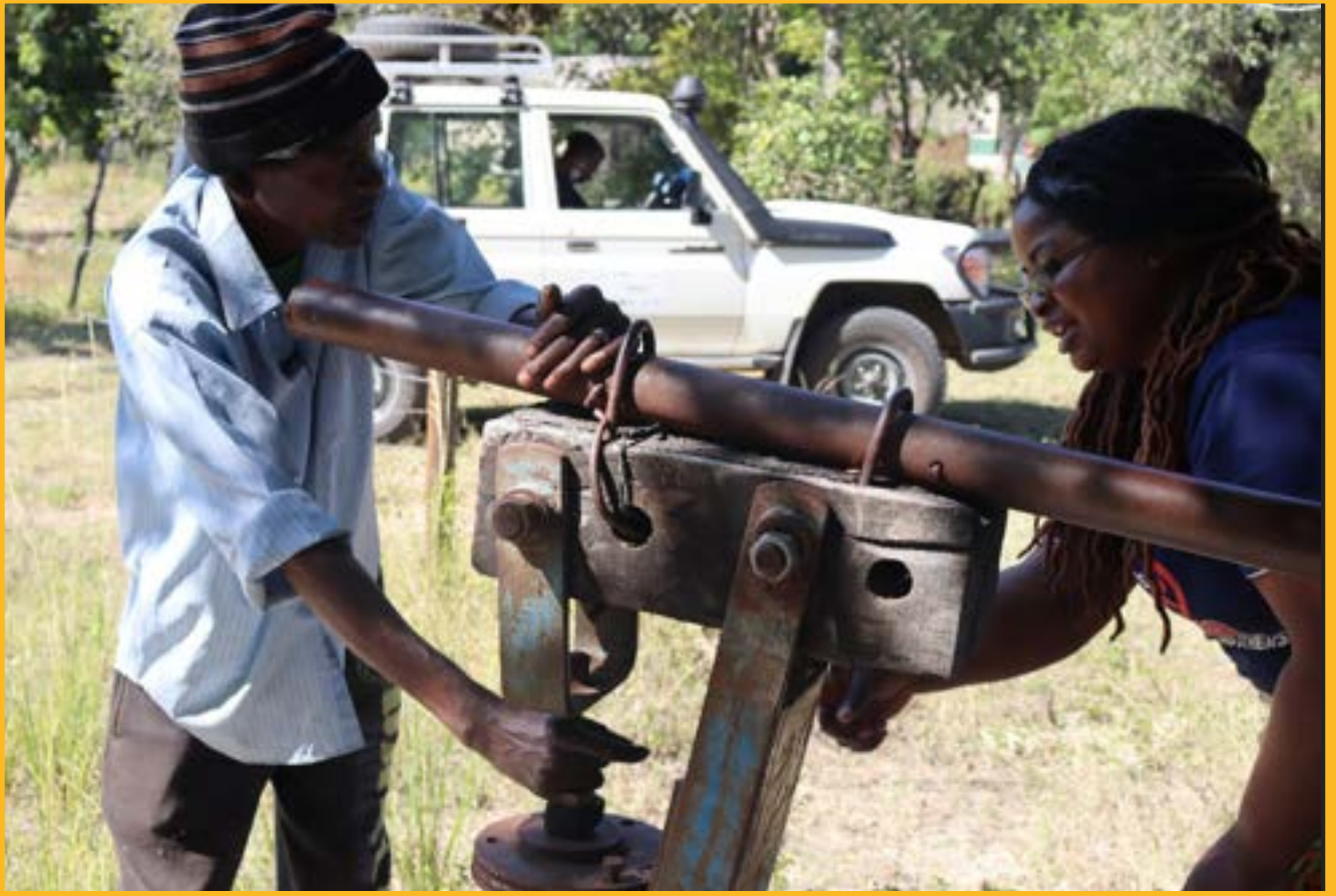
David Mabomhe, a Village Pump Minder in Ringai village and Takunda Mutare WASH Officer assessing a borehole in Ward 12. Takunda is rehabilitating non-functional boreholes for the communities to access portable drinking water. © Kudakwashe Murambadoro/ TAKUNDA RFSA
